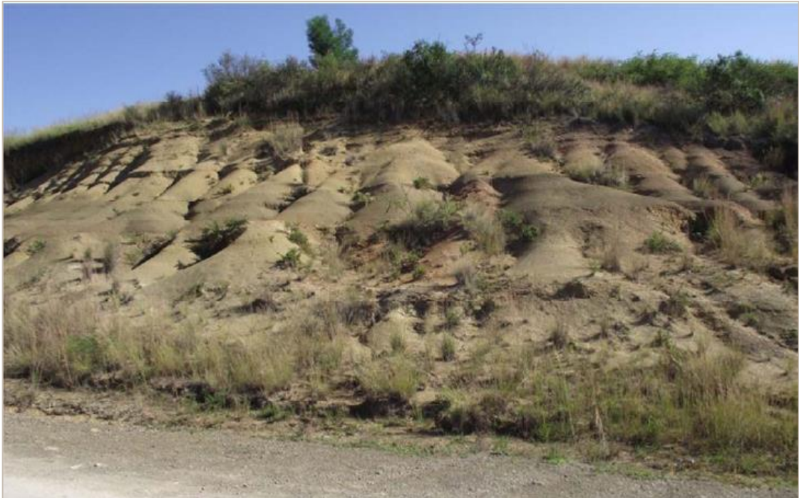
Figure 4.9: Erosion associated with the road network in the Luhane catchment
