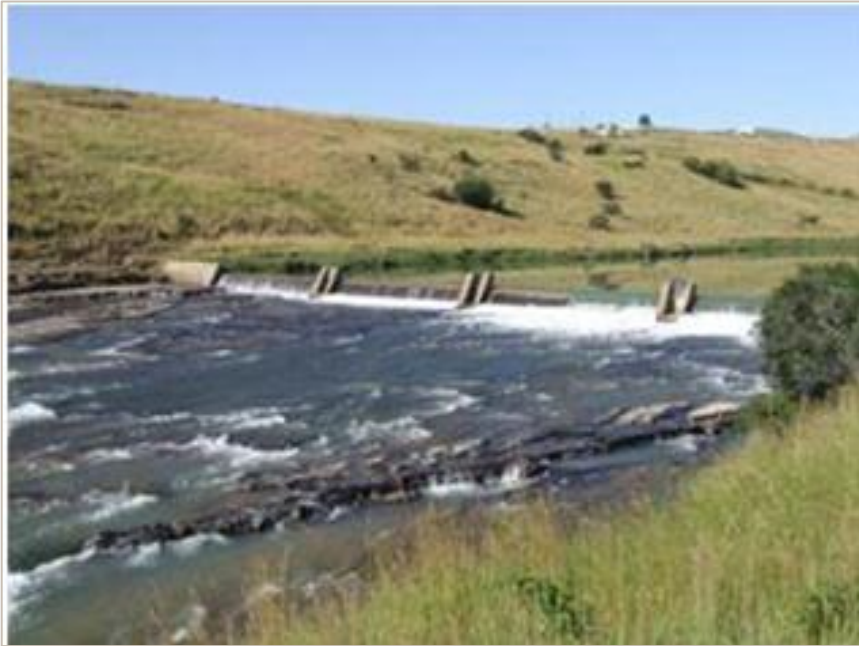
Figure 5.1: Sample point at uMkhomazi River at Lundy's Hill weir
