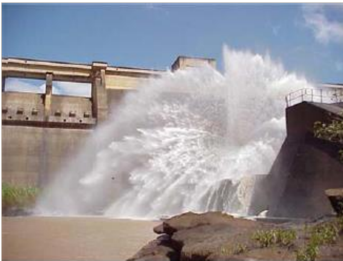
Figure 6.1: Sleeve valves reoxygenate water released from Hazelmore dam
