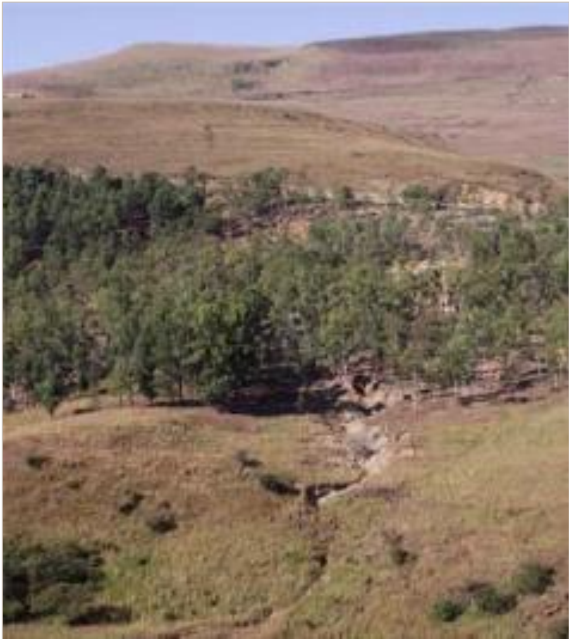
Figure 4.14: Alien invasive tree woodlot associated with significant erosion
